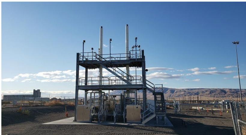
*EM’s Office of River Protection and tank operations contractor Washington River Protection Solutions continue to enhance safety in the Hanford Site’s Tank Farms with the completion of a new exhauster ventilation system in the SY Tank Farm. All six of Hanford’s double-shell-tank farms are now ventilated by upgraded exhauster systems.*
