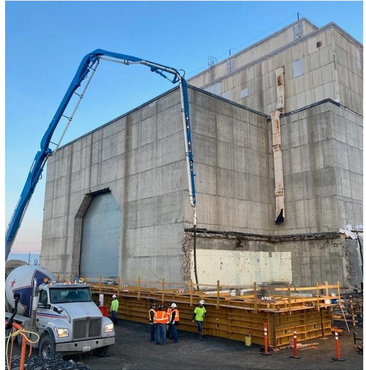
*Workers with EM contractor Central Plateau Cleanup Company pour concrete for a 6-foot-thick foundation to support a massive steel structure over the former K East Reactor building. The enclosure is designed to protect the building while the radioactivity in the reactor core decays over the next several decades, making it safer and easier to complete disposition of the reactor in the future. The project is one of EM’s top construction priorities for 2022.*
