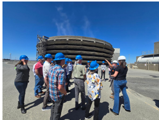
Cooling Towers at Energy Northwest
