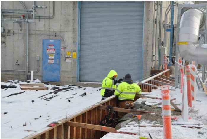
Jason Beaver and Pedro Ramirez with EM Richland Operations Office contractor Central Plateau Cleanup Company construct wooden forms for a new concrete pad outside the Waste Encapsulation and Storage Facility where trucks will pick up casks filled with radioactive capsules for the short trip to a nearby dry-storage area.
