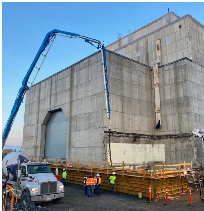
Workers with EM contractor Central Plateau Cleanup Company pour concrete for a 6-foot-thick foundation to support a massive steel structure over the former K East Reactor building. The enclosure is designed to protect the building while the radioactivity in the reactor core decays over the next several decades, making it safer and easier to complete disposition of the reactor in the future. The project is one of EM’s top construction priorities for 2022.
