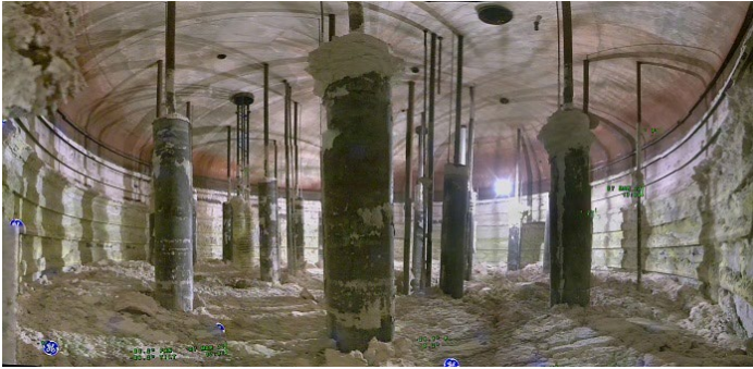
Waste retrieval from Tank AX-101, the last of four tanks to be retrieved in the Hanford Site's AX Farm, is set to begin this fall. This in-tank photo shows the salt-based waste and the tank's 22 air-lift circulators.
