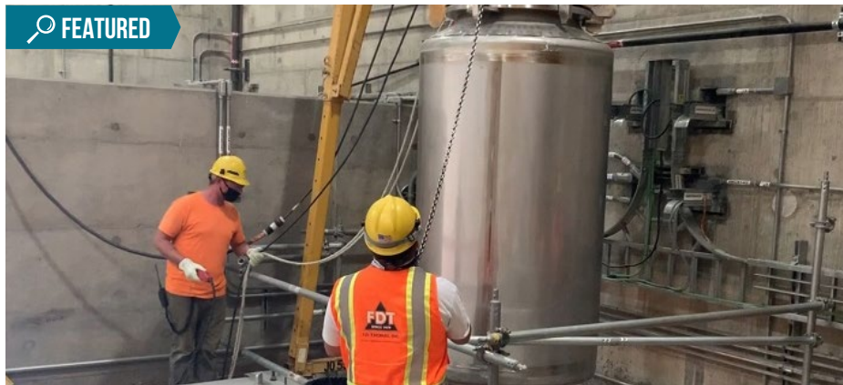
Workers at the Hanford Waste Treatment and Immobilization Plant test the Low-Activity Waste Facility's container handling system.
