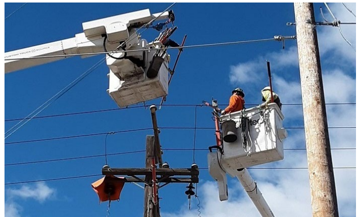
Crews updated Hanford's massive electrical system, replacing miles of electrical lines, and adding fiber optic communication cables and new utility poles as part of infrastructure upgrades in support of the Direct-Feed Low-Activity Waste Program.
