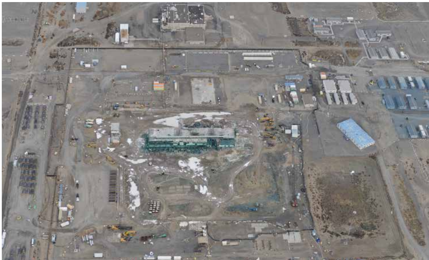
Higher-risk demolition work will start up again at the PFP shortly.
