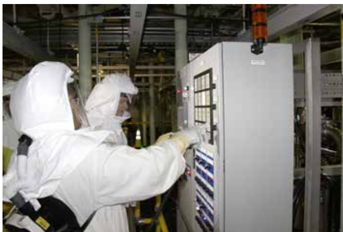
Workers are using innovative technology to remove sludge from the K West Basin.
