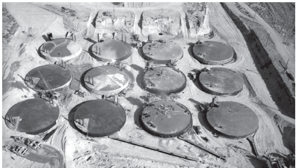
The external structure of Hanford's underground storage tanks, shown here during construction more than 50 years ago, was recently deemed “good” by an independent qualified registered professional engineer.
