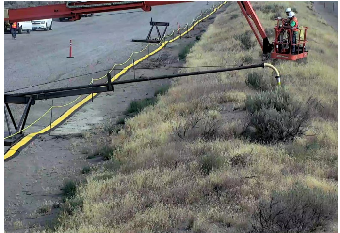
Workers filled Tunnel 2 near the Plutonium Uranium Extraction Facility with engineered grout to prevent it from collapsing.
