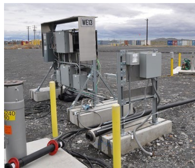
EM contractor Central Plateau Cleanup Company is implementing a new soil flushing system near the Hanford Site’s former K East Reactor. The system forces residual chromium contamination in the soil down to groundwater, where it will be extracted through a network of existing wells and sent to a nearby treatment facility.
