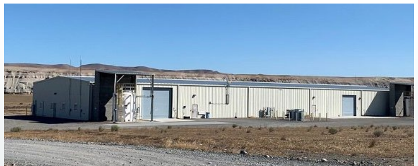
The 100-HX Pump-and-Treat Facility is one of five treatment facilities that removes contaminants from groundwater along the Columbia River at Hanford.
