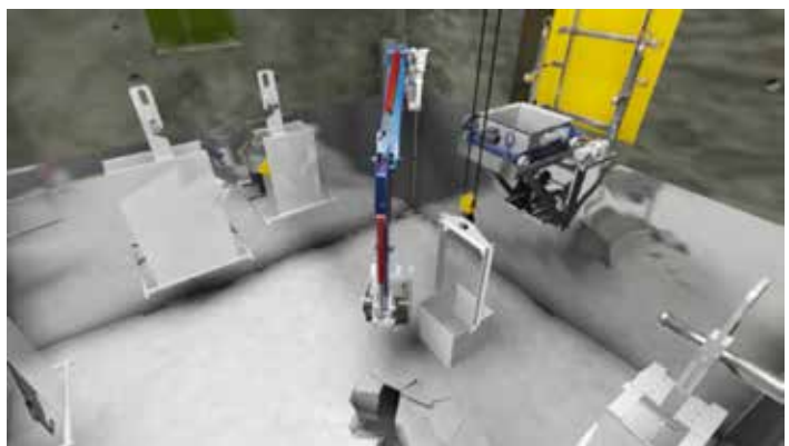
This conceptual illustration shows the remote-operated excavator and load-out mechanism to remove contaminated soil from beneath Building 324.
