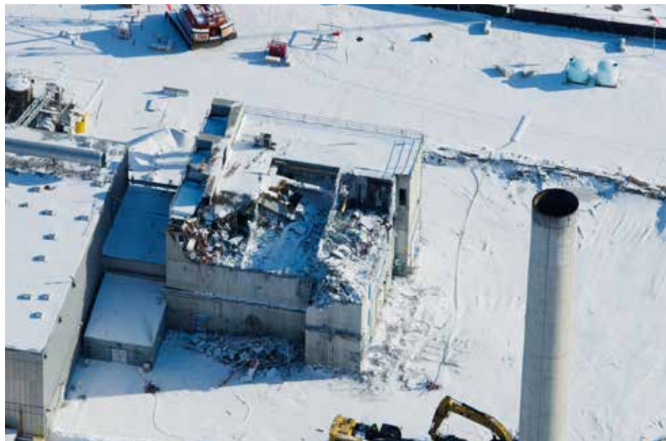
An aerial view of PFP shows a snowy and partially-demolished fourth floor of the Plutonium Reclamation Facility.
