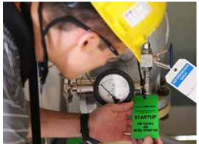
Workers tagged equipment for turnover to startup for testing.
