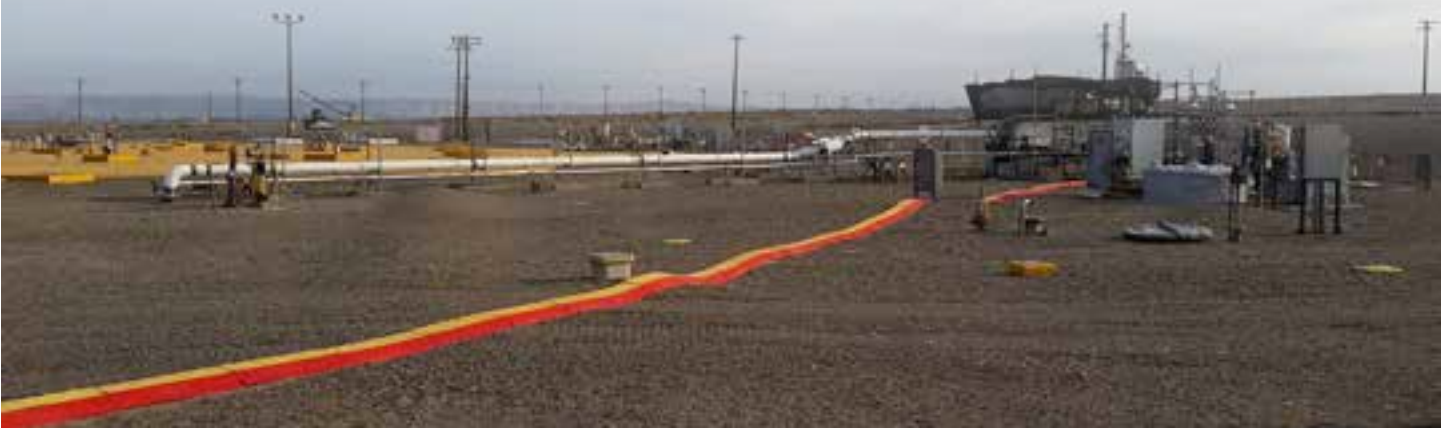
Workers are using a portable exhauster to remove excess liquid from Tank T-111, which is considered to be leaking.
