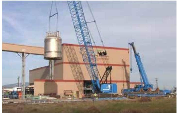
Cranes remove a 30-ton vessel from the WTP Full-Scale Vessel Test Facility to make way for the larger, final vessel.
