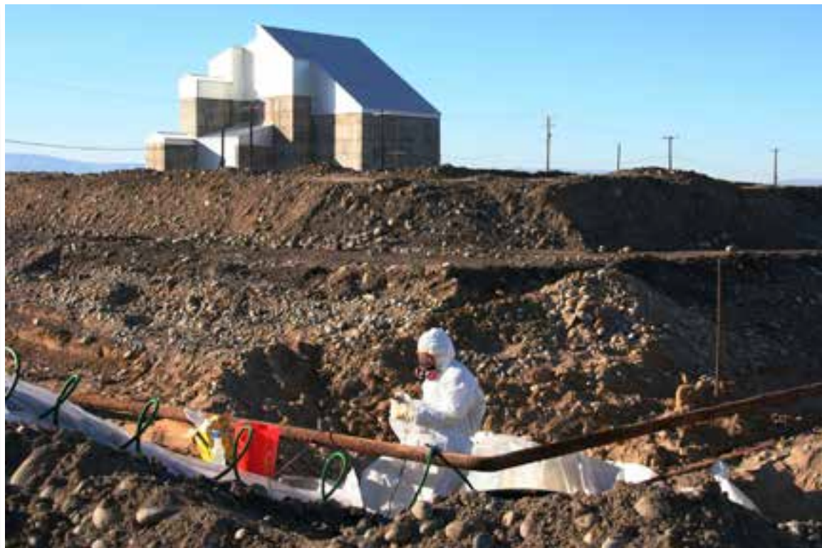
Workers drained pipes below the 100-F area as part of efforts to remove chromium-contaminated soil near the Columbia River.
