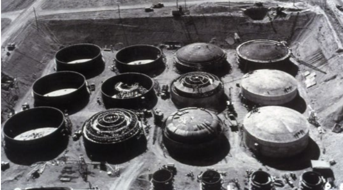
Hanford's B Tank farm under construction during World War II. There are a total of 177 single-shell and double-shell tanks at Hanford, well past their design life and holding 56 million gallons of radioactive and chemical waste.
