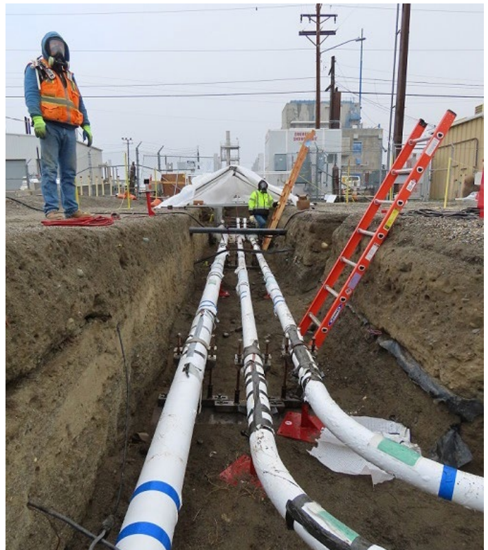
Crews installed double-walled pipes on the Hanford Site as part of the project to replace older transfer lines between waste storage tanks and the 242-A Evaporator.
