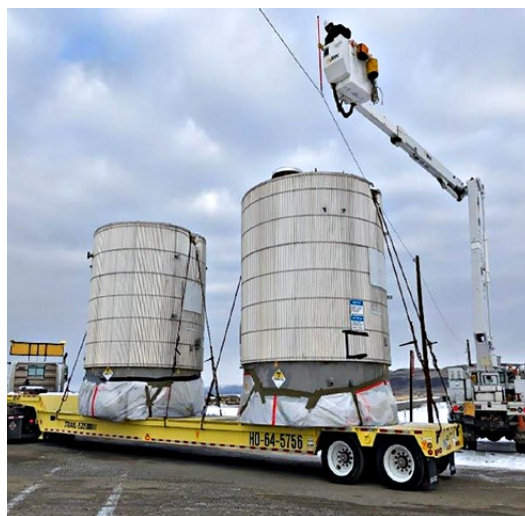
Electrical lineworkers with Hanford Mission Integration Solutions carefully lift overhead power lines to allow a trailer hauling empty tanks to Hanford's landfill to pass.
