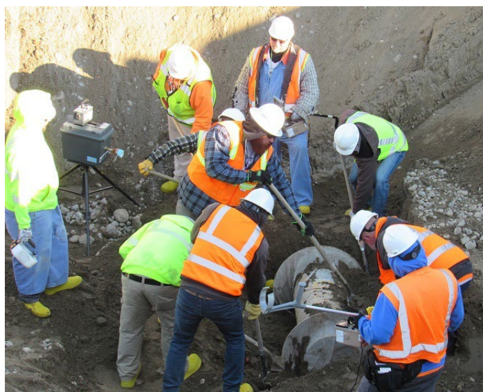
Teams with contractors Central Plateau Cleanup Company and Hanford Mission Integration Solutions recently recovered spent fuel containers from former plutonium production activities on the Hanford Site.
