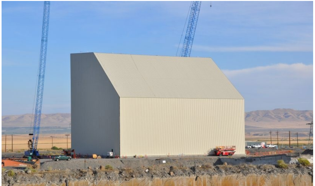
Workers with EM contractor Central Plateau Cleanup Company recently completed construction of a protective enclosure, or cocoon, over the former K East Reactor building. The cocoon is designed to protect the reactor building while the radioactivity in the deactivated reactor core decays over the next several decades, making it safer to complete disposition of the reactor in the future.
