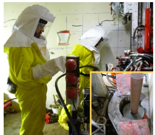
Inside an area of the 324 Building on the Hanford Site, workers recently installed 13 structural supports, called micropiles, to ensure the integrity of the building during the removal of contaminated soil under the facility.
