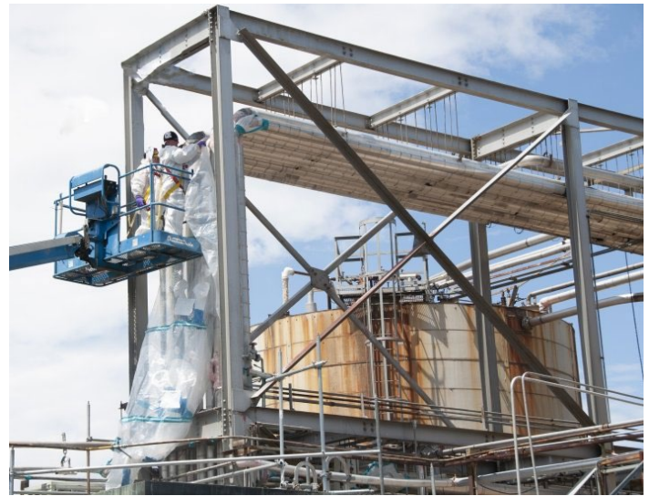
Crews at the Plutonium Uranium Extraction Plant install bags on a piping system to safely remove asbestos-containing material in the 203-A Acid Storage Area.
