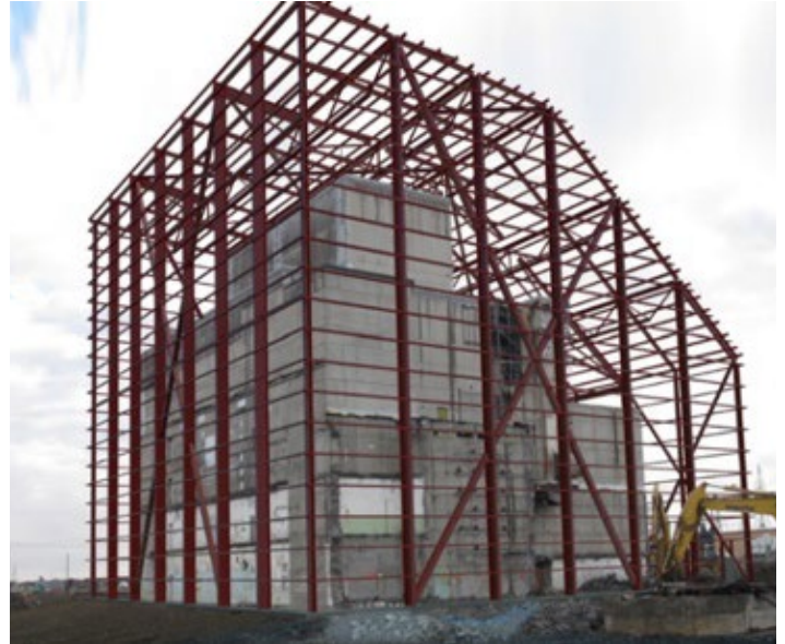
An artist's rendition of the K East Reactor safe-storage enclosure. K East will be the seventh of Hanford's nine former reactors to be placed in interim safe storage while radioactivity in the reactor cores decays over the next several decades, making it easier and safer to dismantle the reactors in the future.
